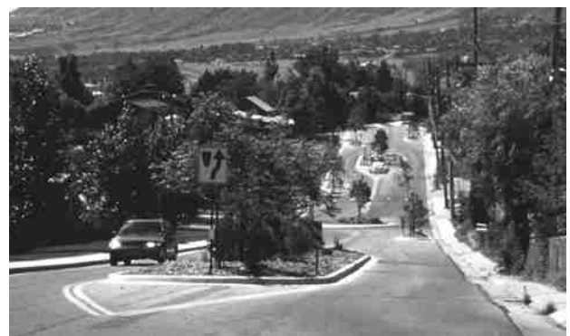
Landscaped medians can effectively reduce the actual and perceived width of a street, thus reducing vehicle speed.
