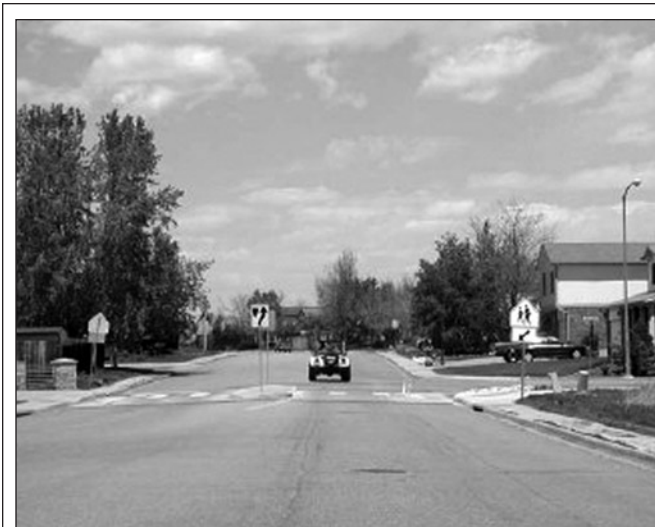
Figure 3a. Raised crossing with a refuge island on Eaton Street.
